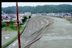
Revetments, Dikes (High Crest)
