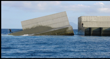
Breakwater damaged by typhoon in 2005 at Higashinohama Port, Kagoshima Pref.
