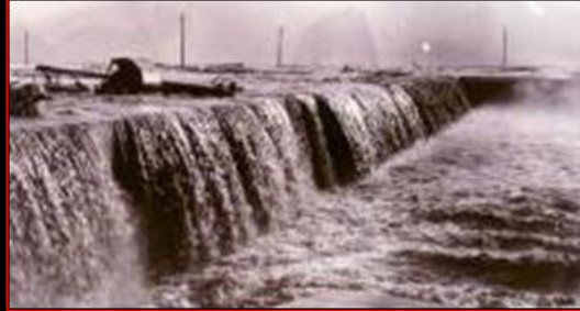
Tsunami overtopping seawall in Iwate Pref. (Chile Earthquake in 1960)
