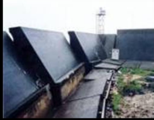
Earthquake caused structural damage
